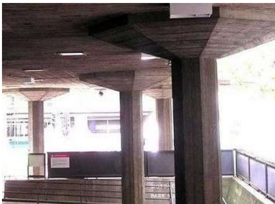
Fig. III Flat slab with a column head
