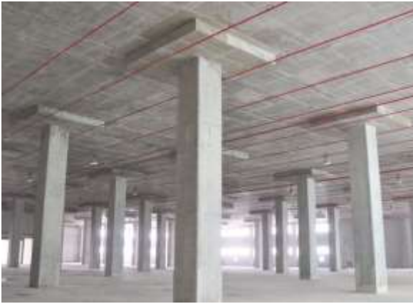
Fig. II Flat slab with drop panels
